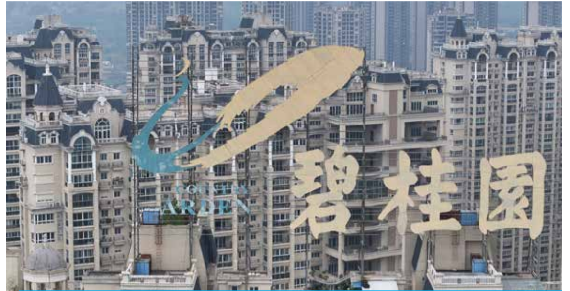
ZHENJIANG, China: This aerial photo taken on October 10, 2023 shows a logo of China's developer Country Garden Holdings on top of a building in Zhenjiang, in China's eastern Jiangsu province. — AFP
