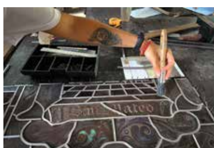
A young participant in an international workshop on stained glass restoration and creation cleans an antique stained glass window.
