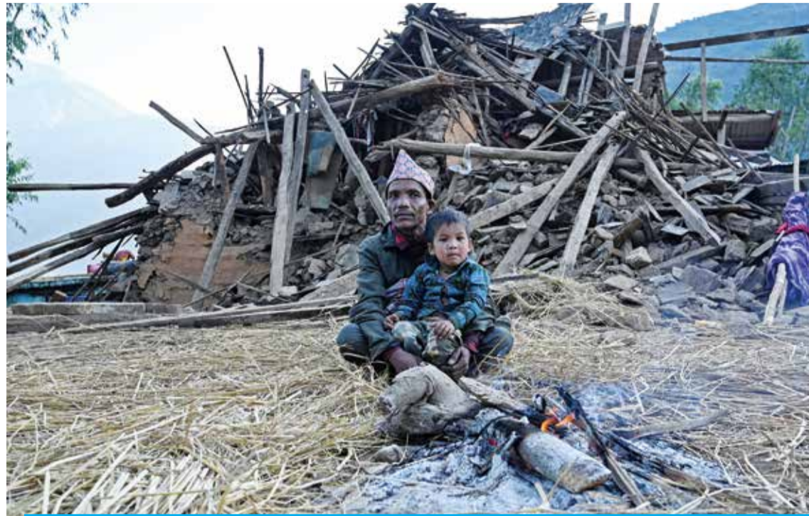
JAJARKOT: Survivors sit in front of a damaged house in Chiuri village at Jajarkot district on Nov 5, 2023. — AFP photos
