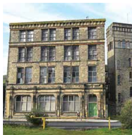
New Mills, a derelict former textile mill in the centre of the village of Marsden.
