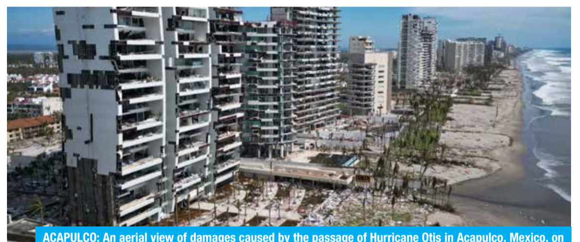
ACAPULCO: An aerial view of damages caused by the passage of Hurricane Otis in Acapulco, Mexico, on Oct 28, 2023. — AFP
