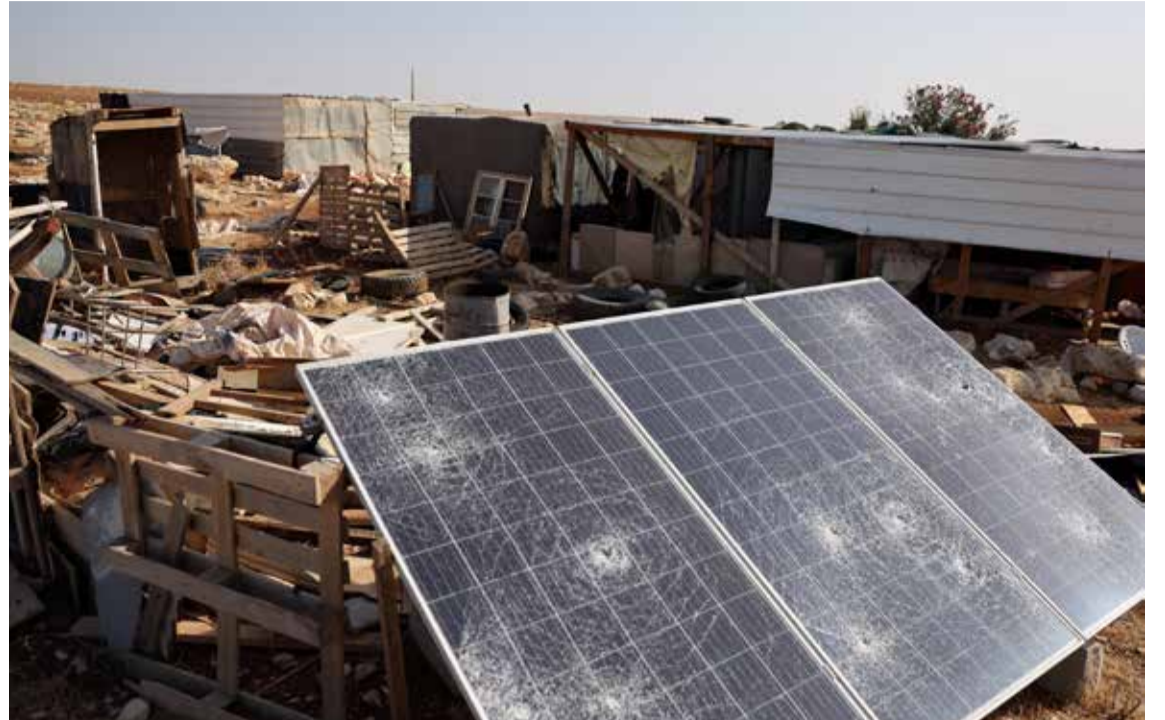
A solar panel is damaged after Zionist settlers attacked the occupied West Bank village of Wadi al-Seeq.
