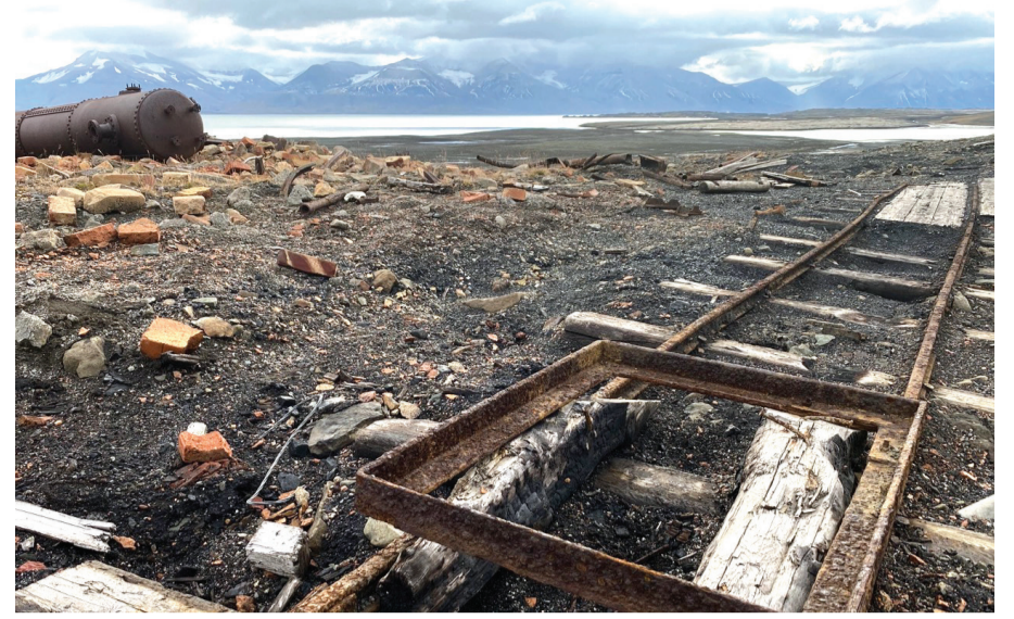
A picture shows rusty railway and rubbles on the site of the former Svea coal mine which operated from 1917 until 2020.
