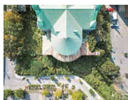
This aerial image shows the exterior of the abandoned Saint-Eusèbe-de-Verceil Catholic Church in the Sainte-Marie borough of Montreal.
