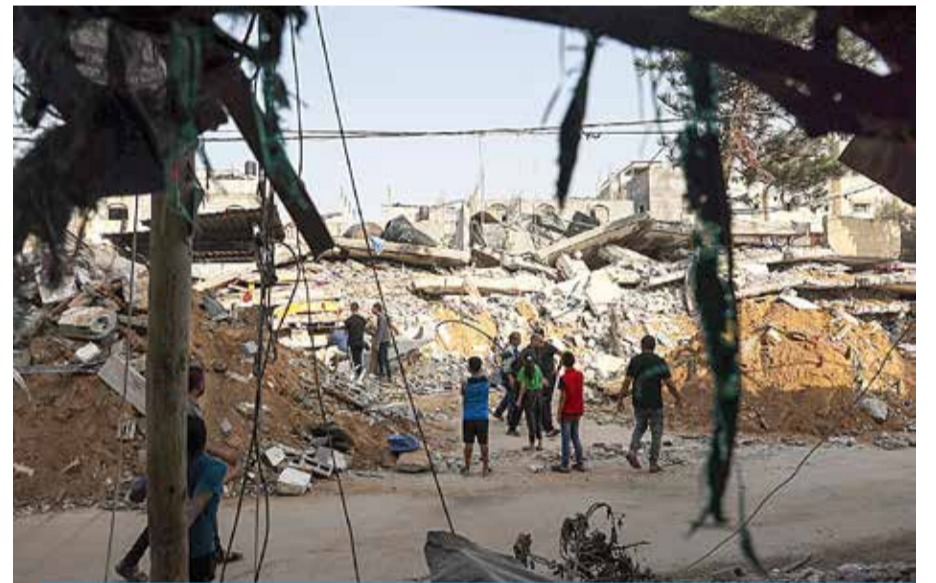
People search the rubble of a building following Zionist strikes on Oct 24, 2023.
