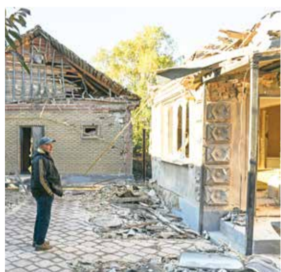
DONETSK: A man stands in the courtyard of his house damaged as a result of a missile strike, in Donetsk on Oct 15, 2023. — AFP
