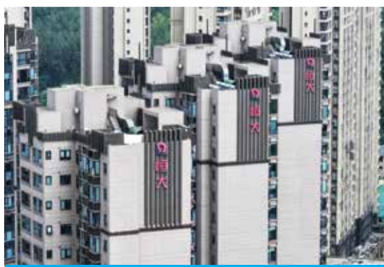
NANJING: The Evergrande logo is seen on residential buildings in Nanjing, in China's eastern Jiangsu province on August 18, 2023. — AFP
