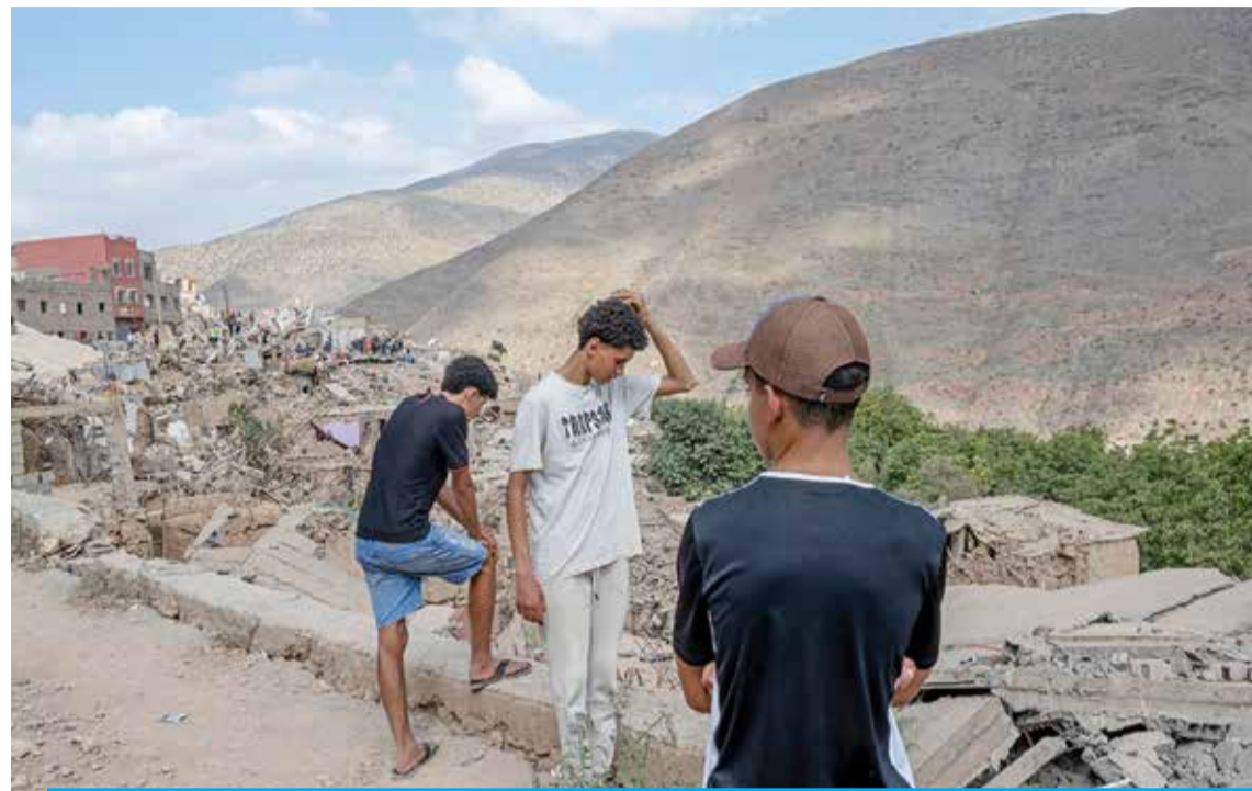
IMI N'TALA: Youths look at the rubble of destroyed houses amid ongoing rescue operations in the village of Imi N'Tala, near Amizmiz, on Sept 12, 2023. — AFP photos
