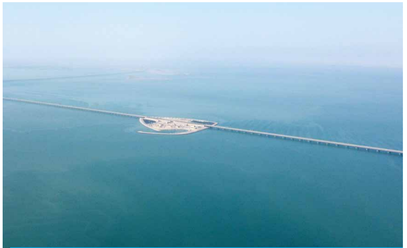
KUWAIT: Photo shows the Sheikh Jaber Causeway in Kuwait City. — Photo by Yasser Al-Zayyat
