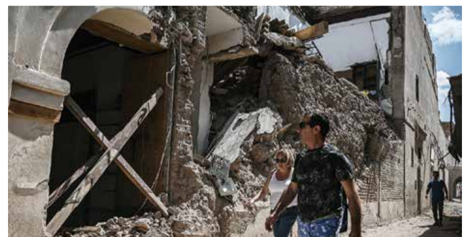
MARRAKESH: Tourists walk past a damaged building in the old quarters of Marrakesh on Sept 12, 2023, following a 6.8-magnitude earthquake. — AFP
