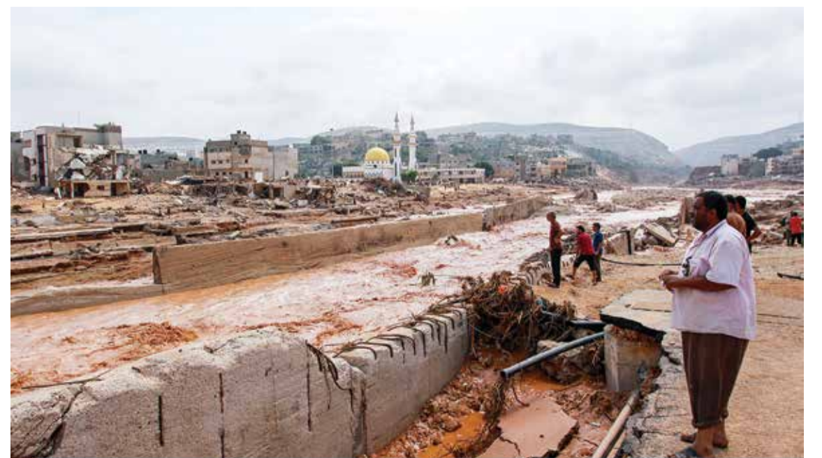
DERNA, Libya: People look at the damage caused by flash floods on Sept 11, 2023. — AFP
