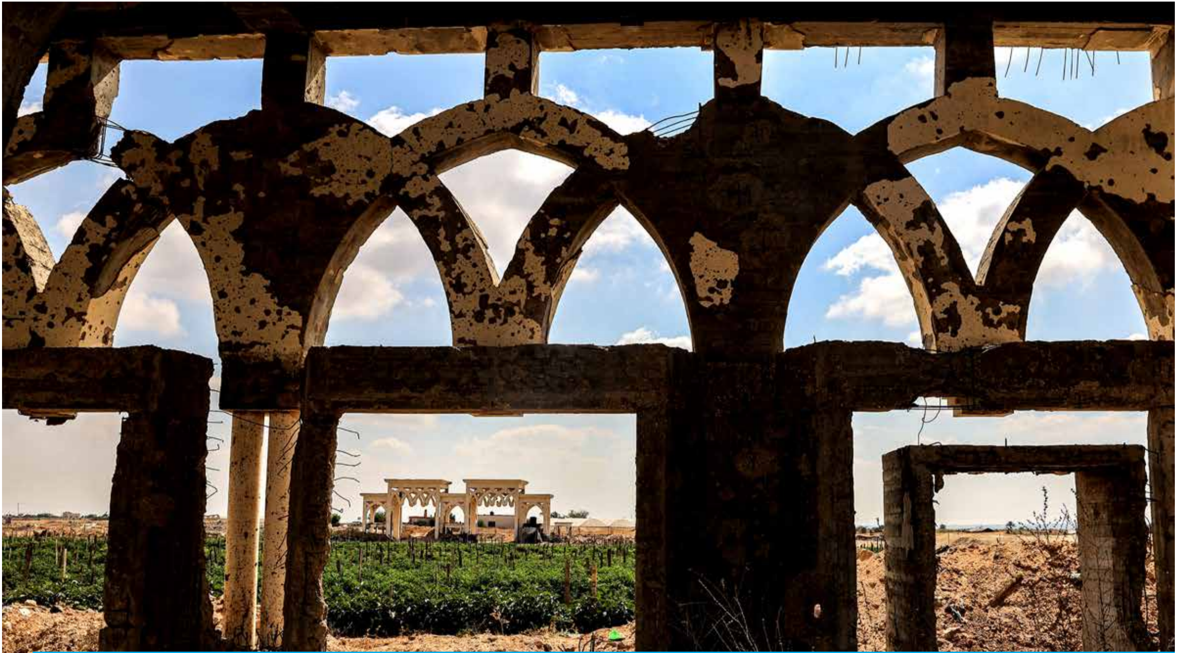
RAFAH: This picture taken on August 27, 2023 shows a view of remaining structures at the destroyed and deserted terminal of the Gaza Strip's former "Yasser Arafat International Airport", in the southern city of Rafah. — AFP
