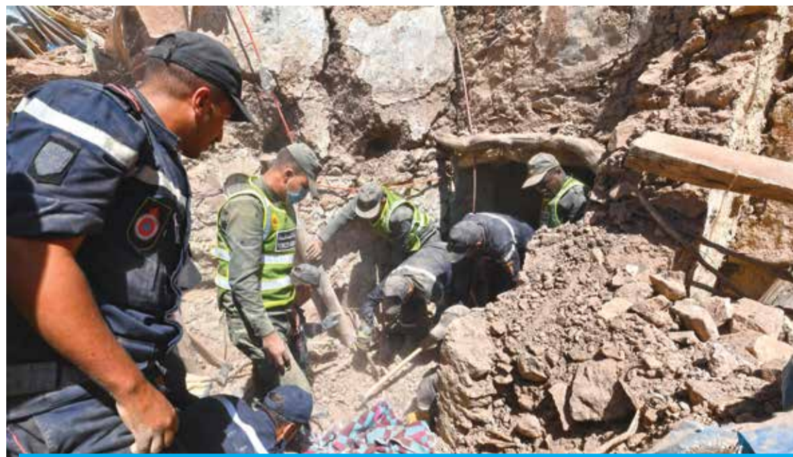
First responders dig in the rubble of the village on September 10, 2023.
