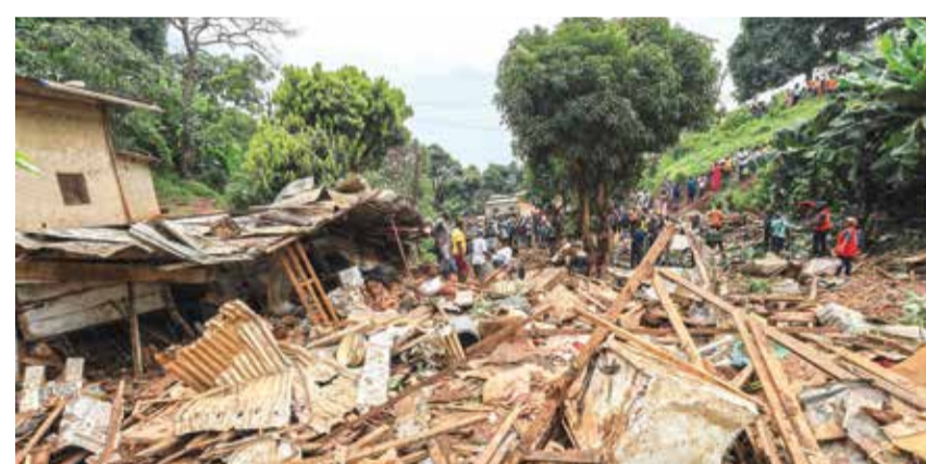
Residents look at the destruction caused by the landslide.
