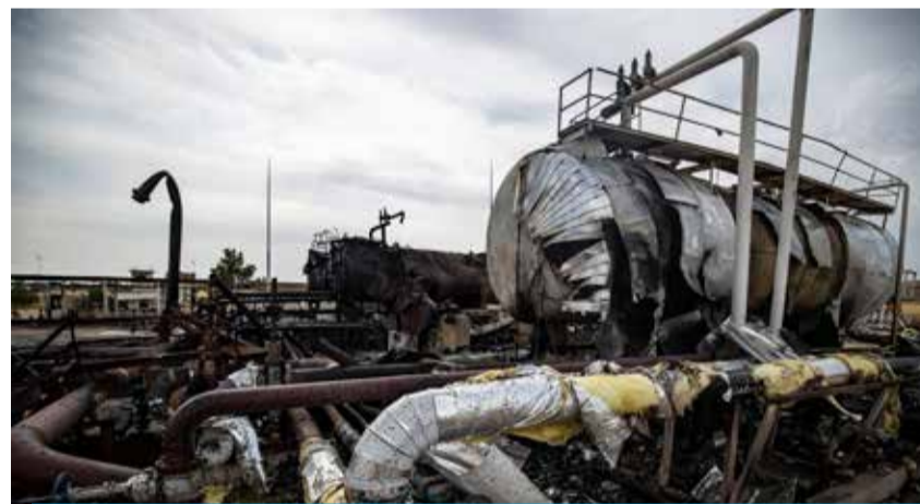
RUMAYLAN: A picture taken on Oct 9, 2023, shows the damage at the Aliyan oil facility in the outskirts of Rumaylan in Syria's Kurdish-controlled northeastern Hasakeh province due to Turkish strikes.
