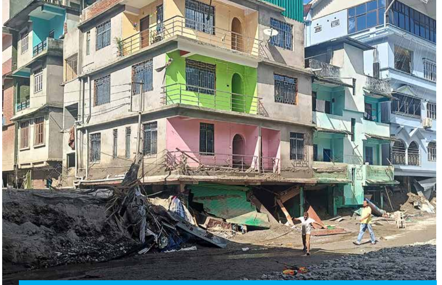
RANGPO: Residents walk along a street covered in mud and debris past damaged buildings on Oct 6, 2023. — AFP
