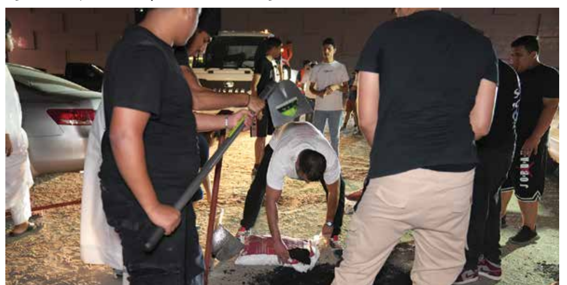
Volunteers help Bu Jarrah fill potholes.
