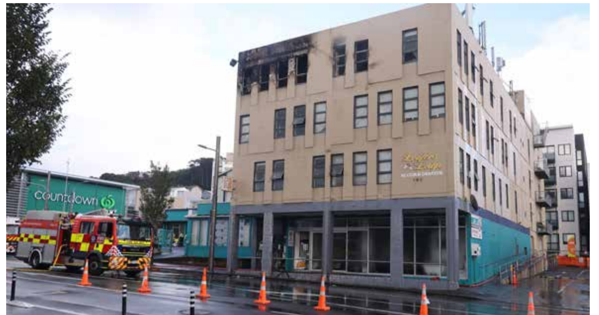
WELLINGTON: Damage is seen on the Loafers Lodge hostel building following a fatal fire in Wellington on May 16, 2023. At least six people have been killed in a fire that erupted in the early hours of Tuesday. — AFP
