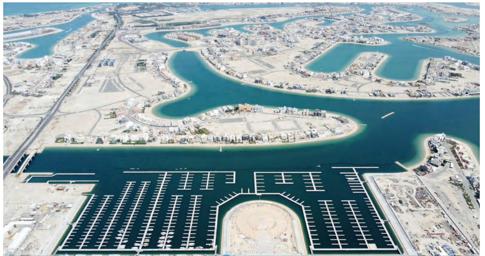
KUWAIT: An aerial view of the Khairan Mall, the biggest outlet mall in the Middle East, in the Sabah Al-Ahmad Sea City some 95 km south of Kuwait City. Khairan is a mixed-use, development located in the heart of the Sabah Al-Ahmad Sea City. The 70,000 square meter multi-use waterfront complex includes a five-star resort, 500 retail stores, tempting restaurants, a shopping mall, two residential towers, one furnished apartment tower, and a 900-berth luxury marina. — Photo by Yasser Al-Zayyat
