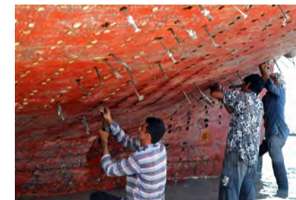
Workers restore a traditional wooden ship (lenj) in a shipyard.
