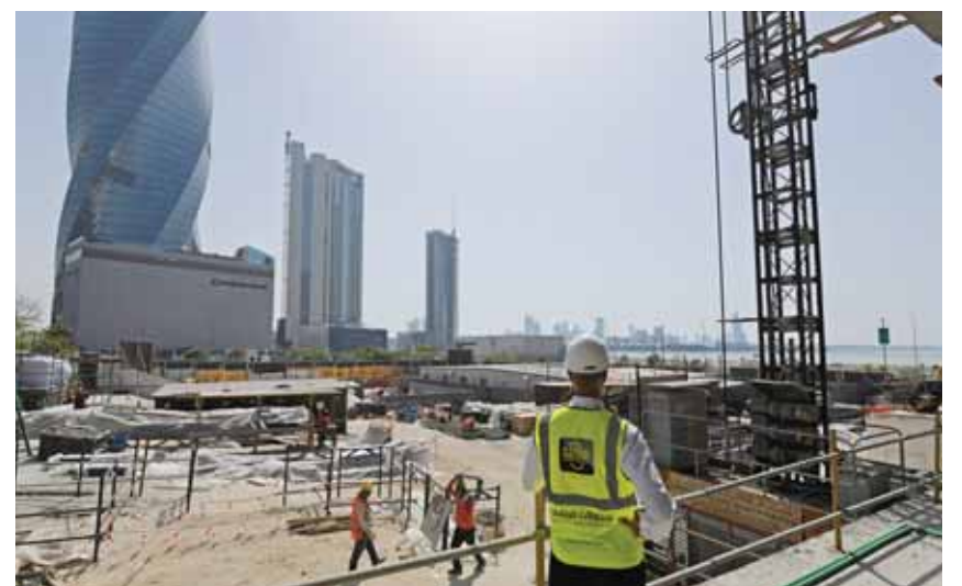
MANAMA: Workers work on the construction site of the Golden Gate towers at Bahrain Bay on March 25, 2023. — AFP
