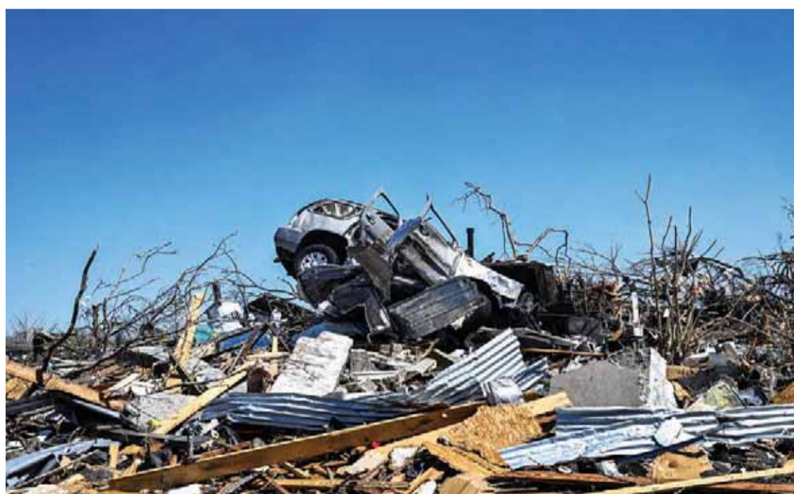
ROLLING FORK: A car sits on top of a damaged house in Rolling Fork, Mississippi, after a tornado touched down in the area, on March 26, 2023. Kuwait Embassy in US has called on Kuwaiti citizens in the southern United States to follow the directives of local authorities as a result of the powerful hurricane that struck the states of Mississippi and Alabama. — AFP
