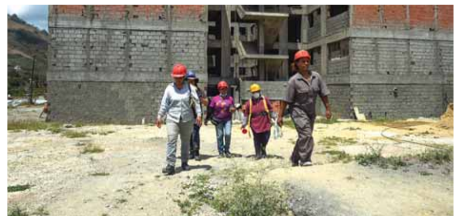
Women workers walk outside the construction of the "Jorge Rodriguez Padre" residential building at lunchtime in the community of Algodonal in Caracas, Venezuela. — AFP photos
