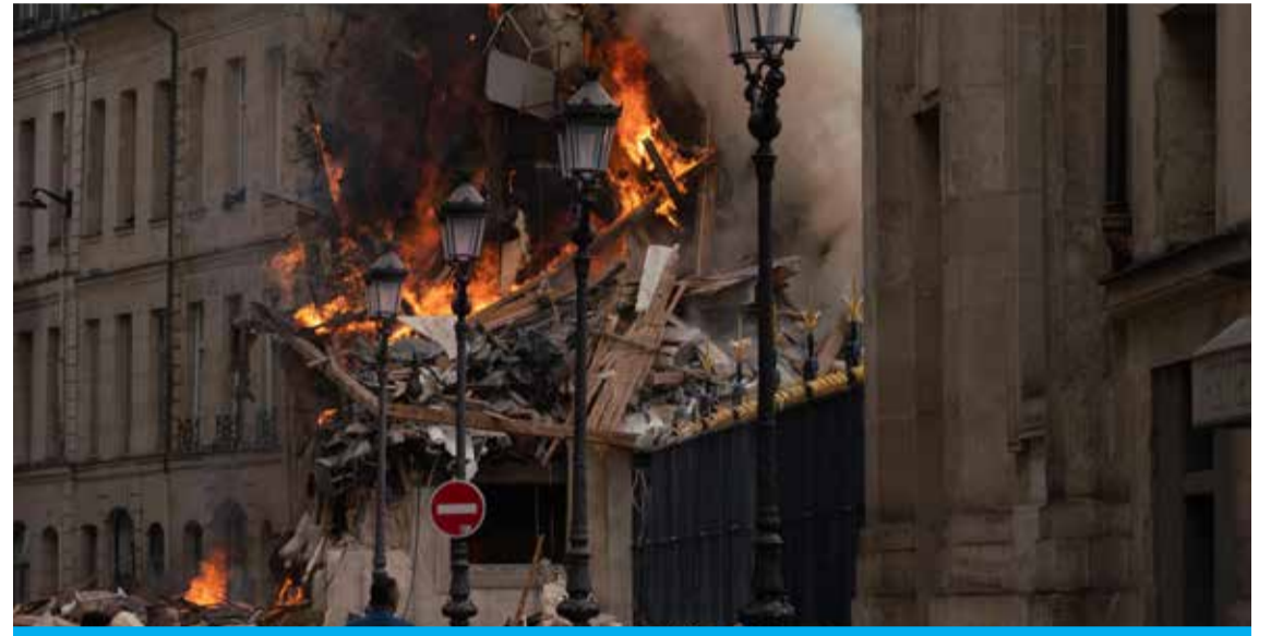
PARIS: Smoke billows from rubbles of a building at Place Alphonse-Laveran in the 5th arrondissement of Paris. A major fire of unknown origin broke out on June 21, 2023 in a building in central Paris, part of which collapsed, injuring 50. — AFP
