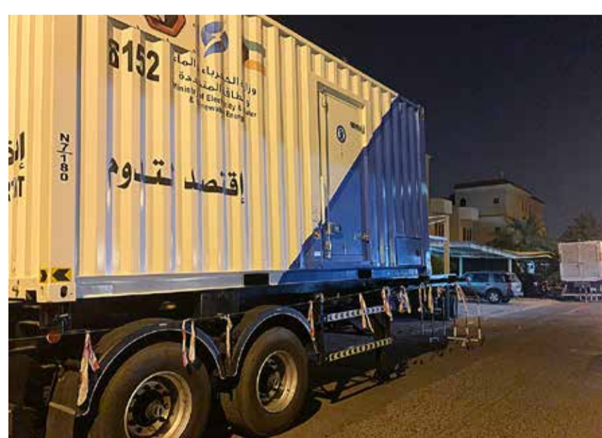
KUWAIT: An emergency team from the ministry of electricity placed generators, seen in the photo, six hours after power was disconnected from a Salwa street on Monday. — Photo by Nebal Snan
