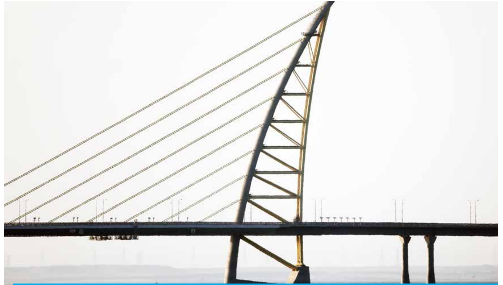
KUWAIT: This photo shows a pylon on the Sheikh Jaber Al-Ahmad Al-Sabah Causeway. The pylon is inspired by the traditional Kuwaiti sailboat and stands at approximately 151 meters, which is about 30 meters higher than the prominent Kuwait Towers. — Photo by Yasser Al-Zayyat
