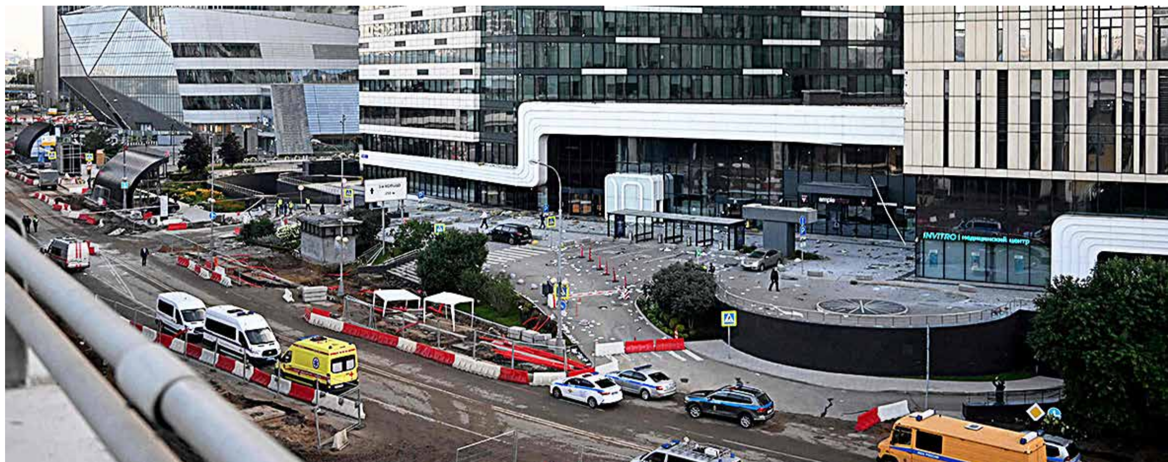
MOSCOW: A view of a damaged office block of the Moscow International Business Center (Moskva City) following a reported drone attack in Moscow on July 30, 2023. — AFP
