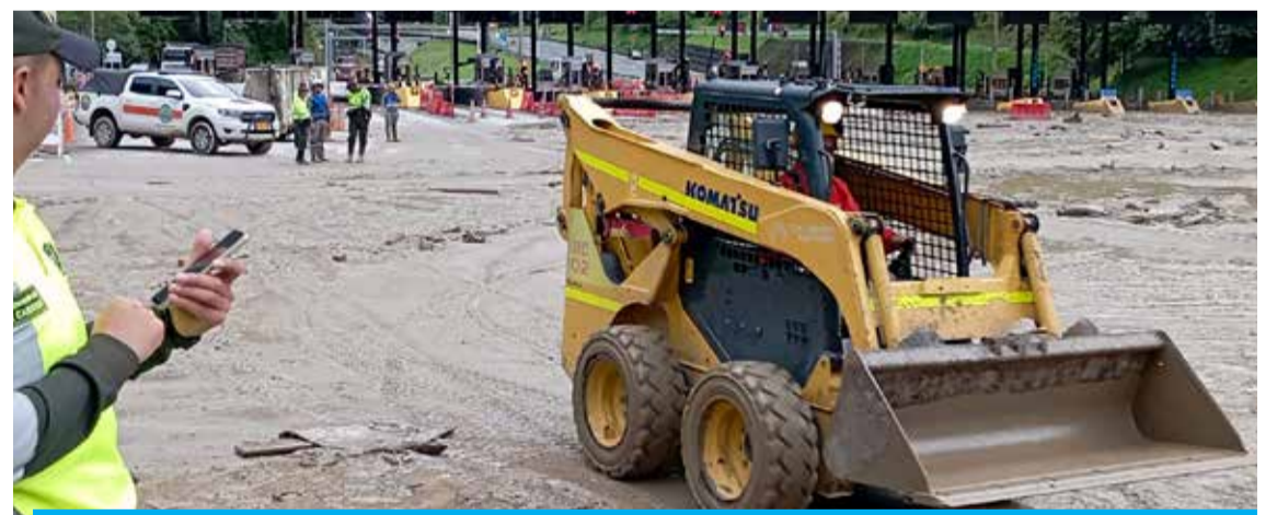
PUENTE QUETAME, Colombia: General view of the Naranjal Toll on the Bogota-Villavicencio highway after a landslide near the town of Puente Quetame, Cundinamarca department, Colombia, on July 18, 2023. — AFP
