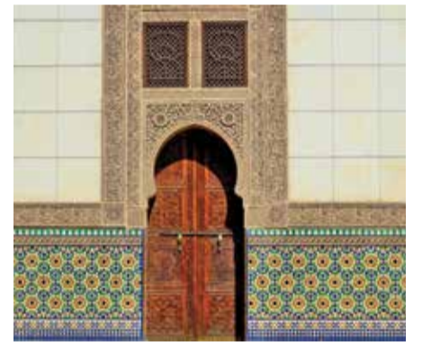
Wooden gate of the building decorated with arabesque designs.
