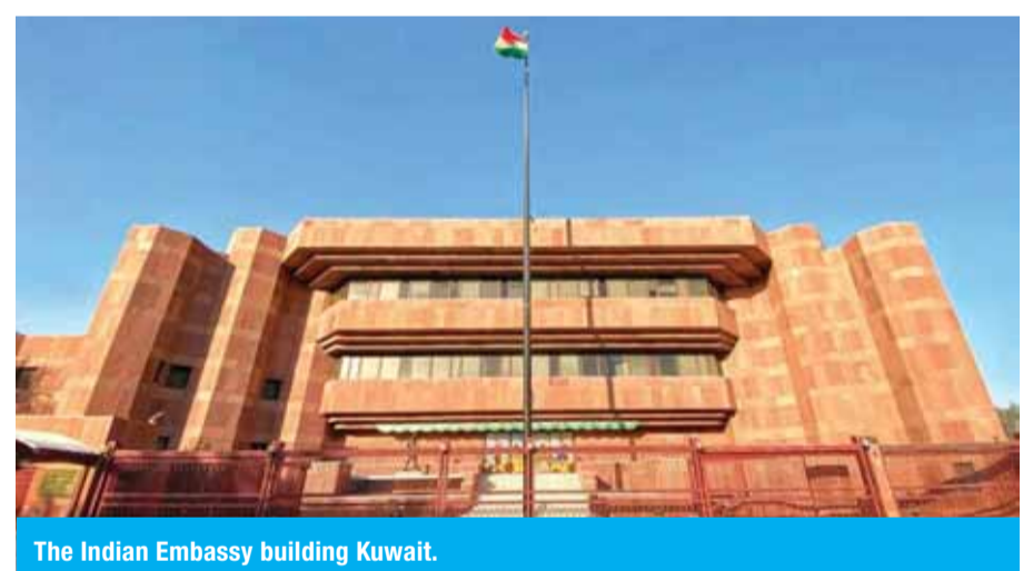
The Indian Embassy building Kuwait.
