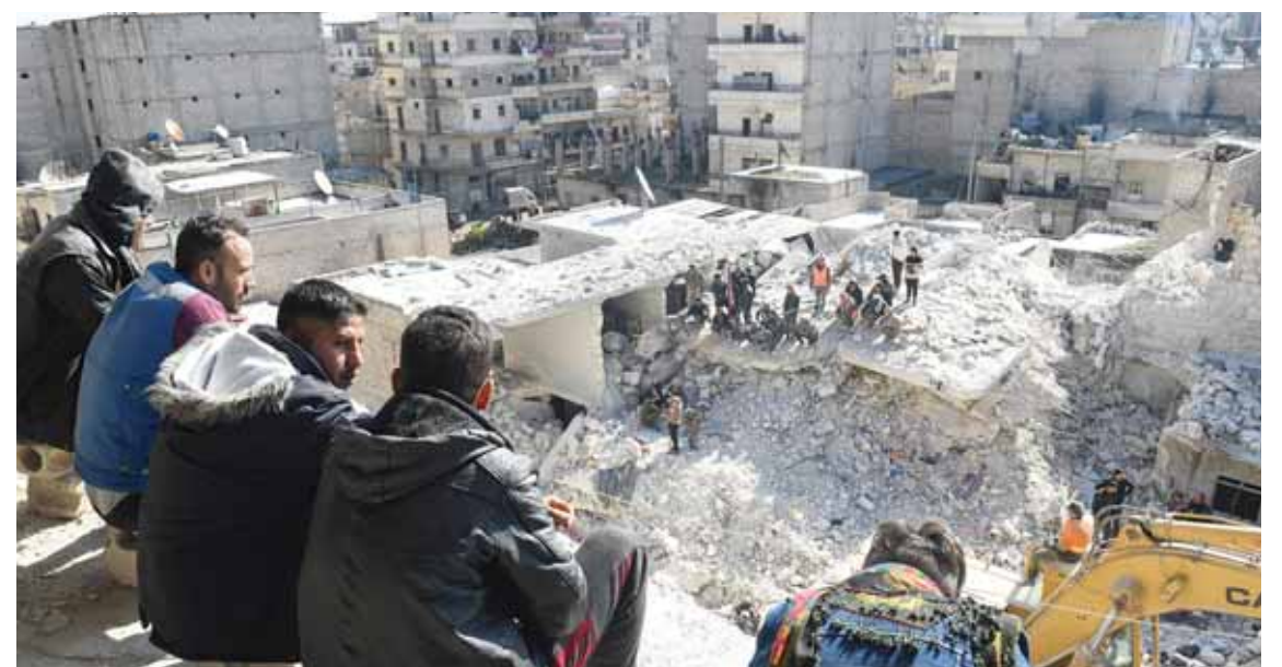
ALEPPO: People watch as rescuers sift through the rubble of a building that collapsed in the northern Syrian city of Aleppo, on January 22, 2023. — AFP
