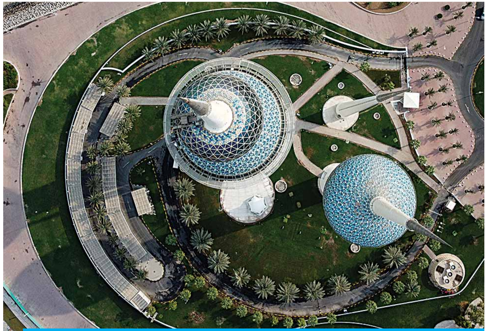
An aerial drone shot of Kuwait Towers on Tuesday. —Photo by Yasser Al-Zayyat
