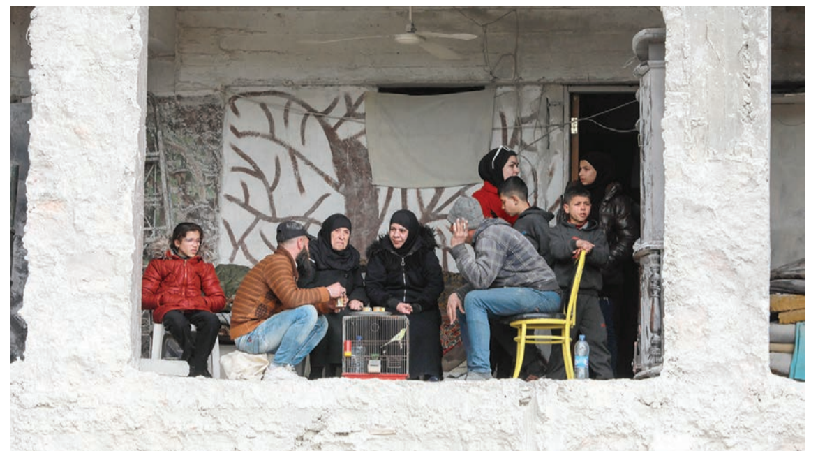
ALEPPO: Ali al-Bash and his mother Amina Raslan drink coffee at home, in a building damaged by the 7.8-magnitude quake, in Aleppo city's al-Masharqa neighbourhood. Aleppo, once a major commercial hub, had already been battered by over a decade of war when the 7.8-magnitude quake struck in early February. —AFP
