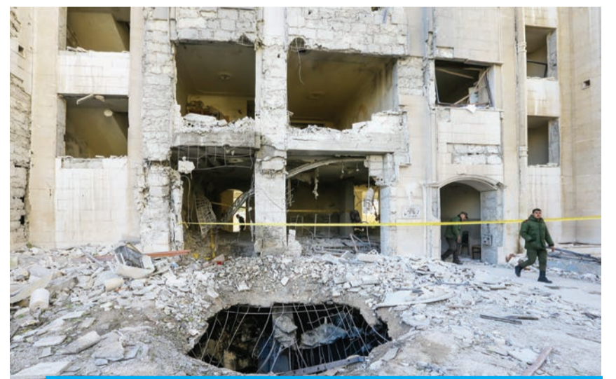
DAMASCUS: Syrian security forces' members inspect a building damaged in a reported Zionist missile strike on Feb 19, 2023. — AFP
