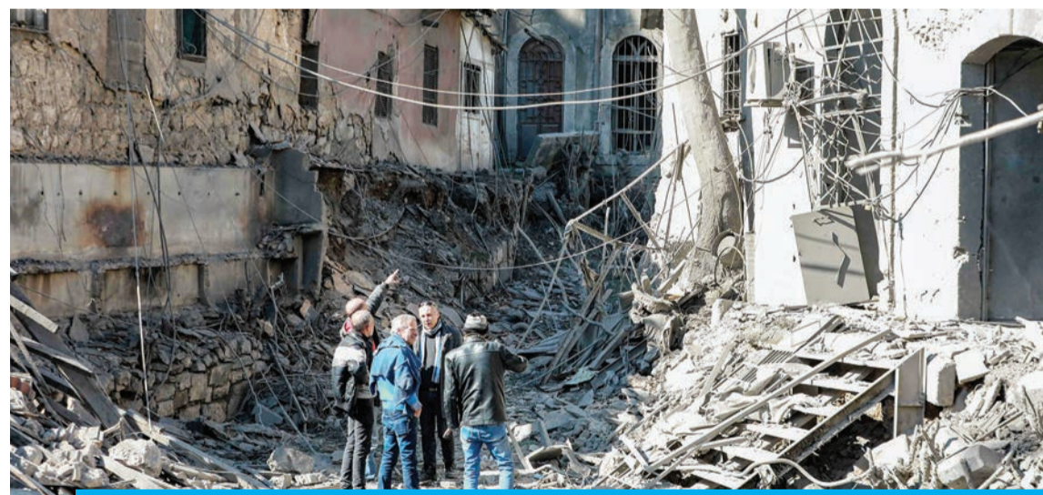
DAMASCUS: People inspect damage in the aftermath of a Zionist air strike that hit the medieval Citadel of Damascus on Feb 19, 2023. — AFP
