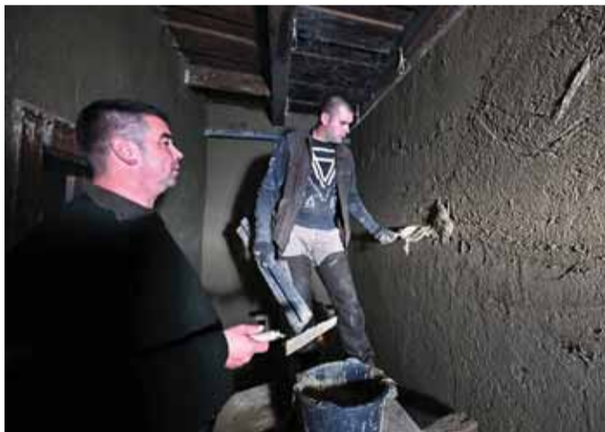
Master builder Janos Gaspar (left) gives instructions to his colleague for mud plaster inside a mud-brick house in Acs.
