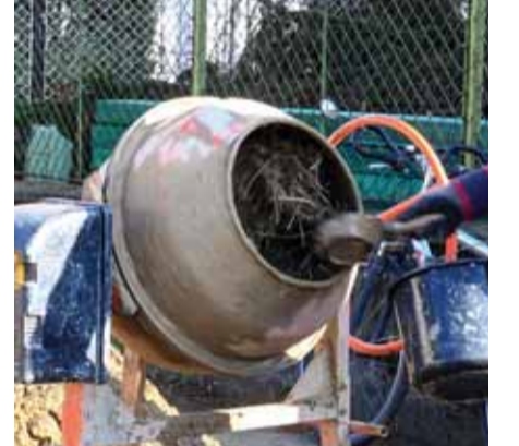
A worker preparing material for the reconstruction of a mud-brick house in Acs.
