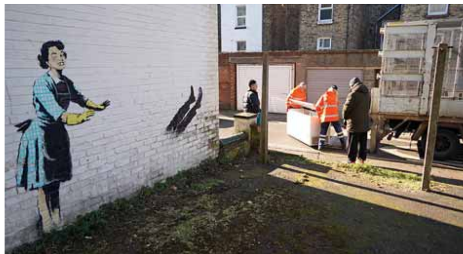
Workers remove a chest freezer that had formed part of an artwork, acknowledge by street artist Banksy, from the side of a house in Margate, south east England. — AFP
