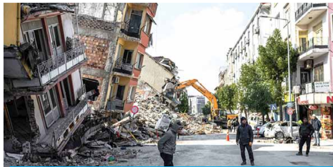
HATAY: People walk next to damaged buildings in the Antakia historical city in Hatay after a 7.8-magnitude earthquake struck the country's south-east. — AFP
