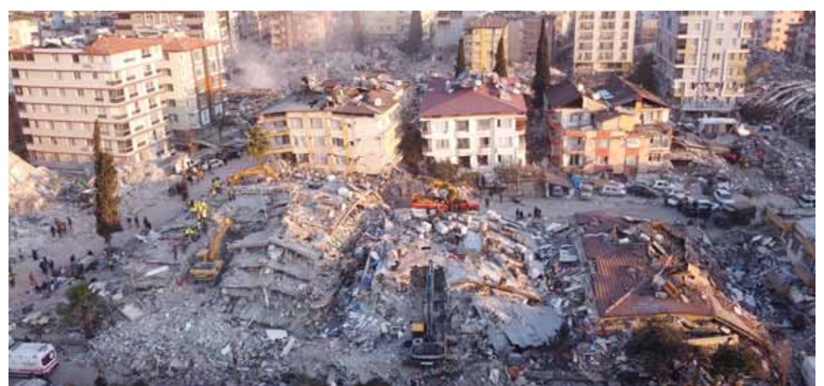
ANTAKYA: An aerial photo shows collapsed buildings in Antakya on February 11, 2023, after a 7.8-magnitude earthquake struck the country's southeast earlier in the week. —AFP
