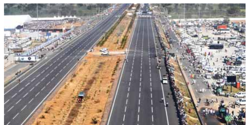
DAUSA, India: People stand along the newly inaugurated Delhi-Dausa-Lalsot section of the Delhi-Mumbai Expressway in Rajasthan on Feb 12, 2023. — AFP
