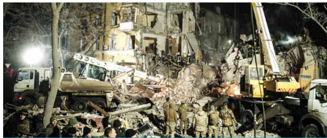
KRAMATORSK: Rescuers remove debris to search for survivors at a destroyed apartment building hit by a rocket in downtown Kramatorsk. — AFP
