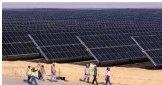
Employees walk at Al Dhafra solar project in Abu Dhabi on Jan 31, 2023. — AFP
