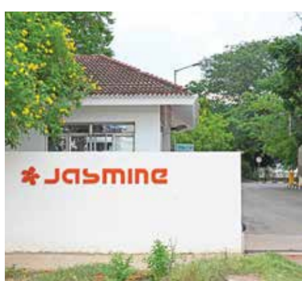
An exterior view of the Jasmine Concrete Exports Private Limited factory in Dindigul.
