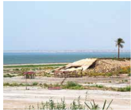
A picture shows dilapidated touristic installations by the Habbaniyah lake affected by severe drought in Iraq's Anbar province.
