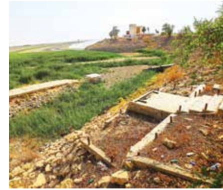
A picture shows dilapidated touristic installations by the Habbaniyah lake affected by severe drought in Iraq's Anbar province.
