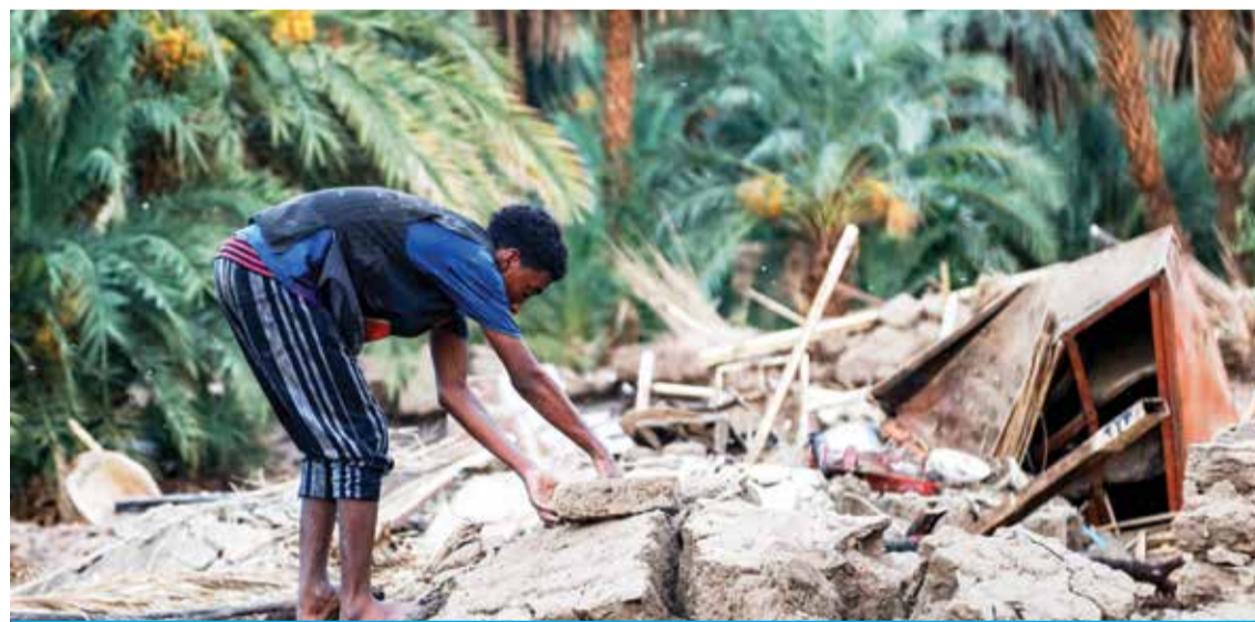
SAQQAI: A man inspects items in the rubble of a destroyed mudbrick house in the aftermath of a flood in al-Sagai north of Omdurman in Sudan on August 6, 2023. — AFP
