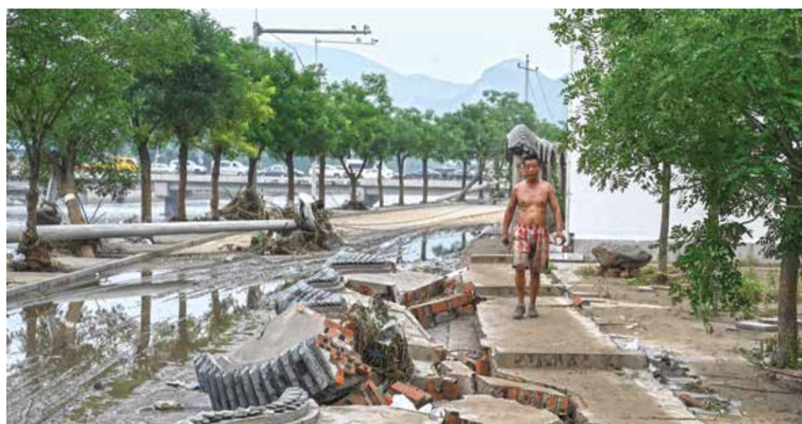
BEIJING: A local resident walks on a broken wall in the aftermath of the flooding at a village following heavy rains in Beijing on August 3, 2023. - AFP
