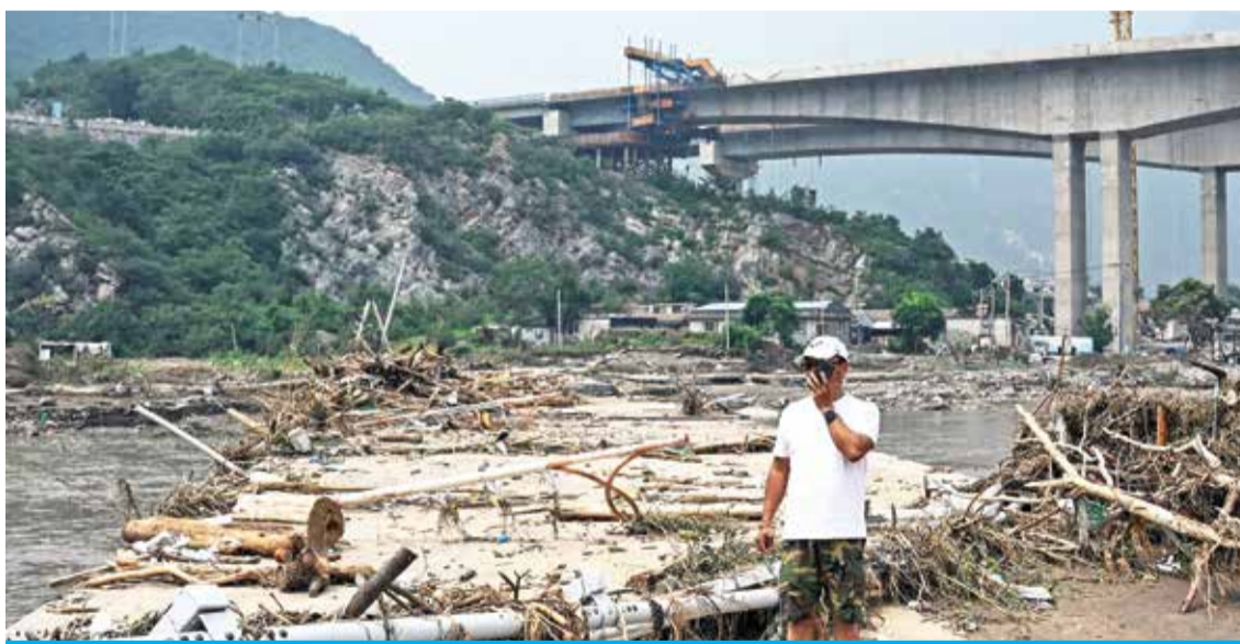
BEIJING: A man stands on a broken bridge in a flood-affected area following heavy rains on Aug 3, 2023. — AFP
