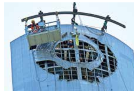
A steeplejack looks out of an opening after the coat of arms of the former Soviet Union from the shield of a 62-meter (102 meters with pedestal) Motherland Monument was removed in Kyiv. — AFP photos
