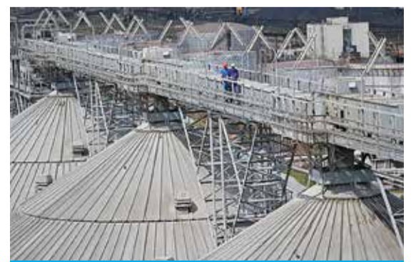
CONSTANTA, Romania: Workers inspect the grain silos at "COMVEX" grain terminal in Constanta harbor, Romania on July 31, 2023.—AFP
