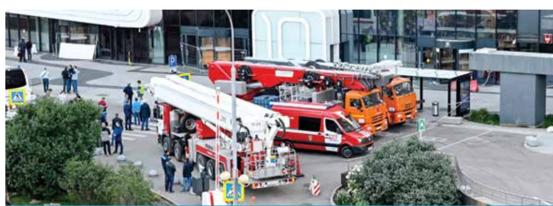
MOSCOW: Emergency personnel work outside a damaged office block of the Moscow International Business Center (Moskva City) following a reported drone attack in Moscow on August 1, 2023. — AFP
