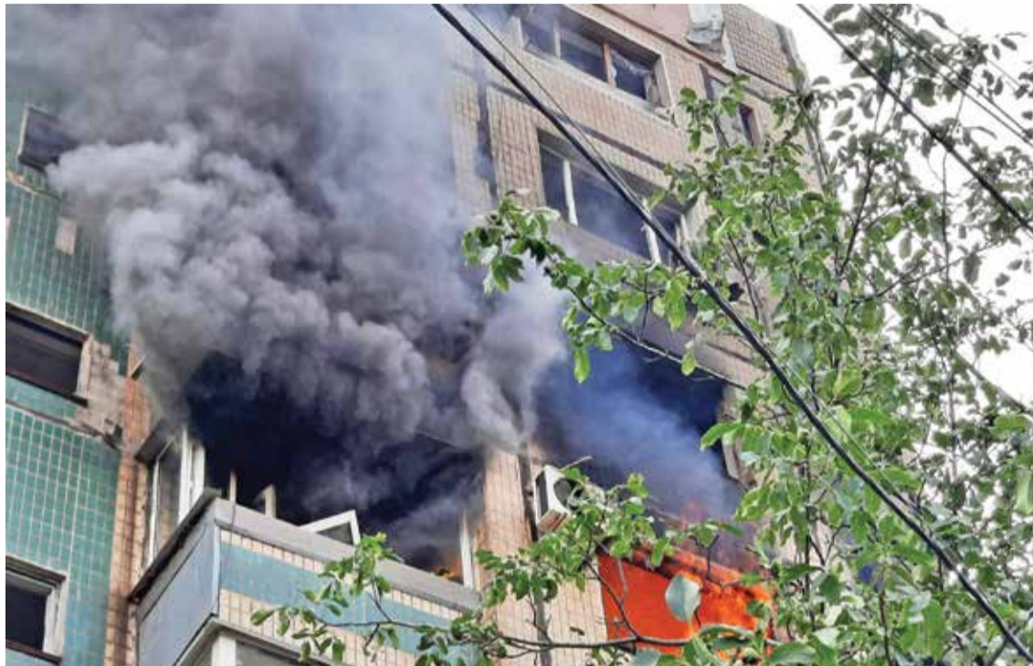
KRYVYI RIG: Fire engulfs a nine-storey residential building partially destroyed as a result of Russian missile strike in Kryvyi Rig, amid the Russian invasion of Ukraine. - AFP
