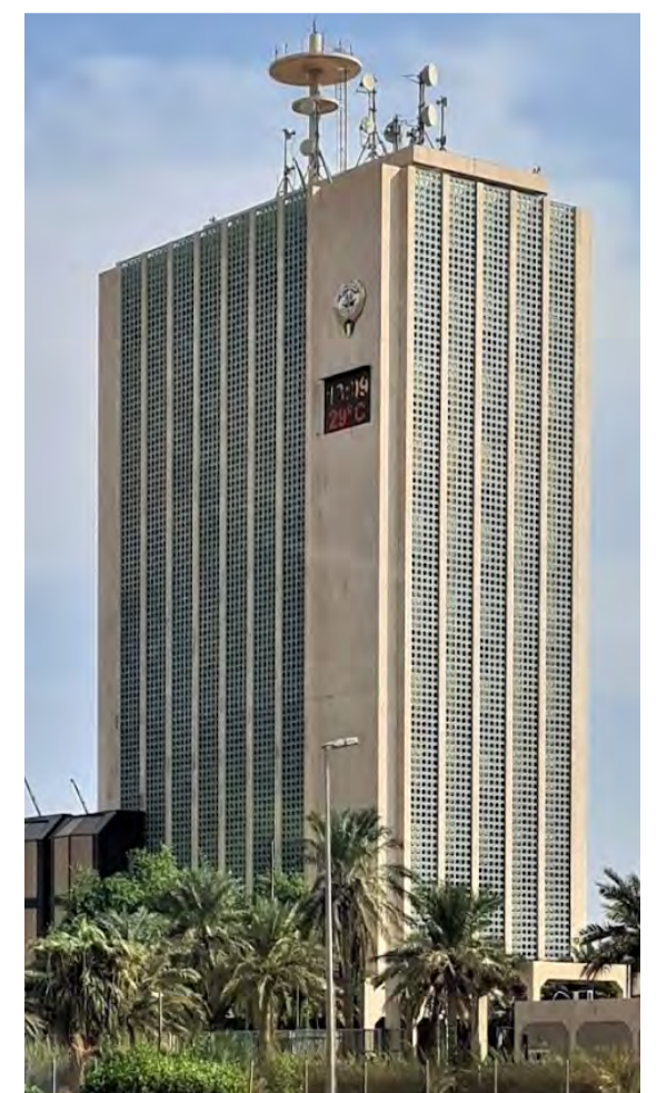
Kuwait's Ministry of Water and Electricity control center.
