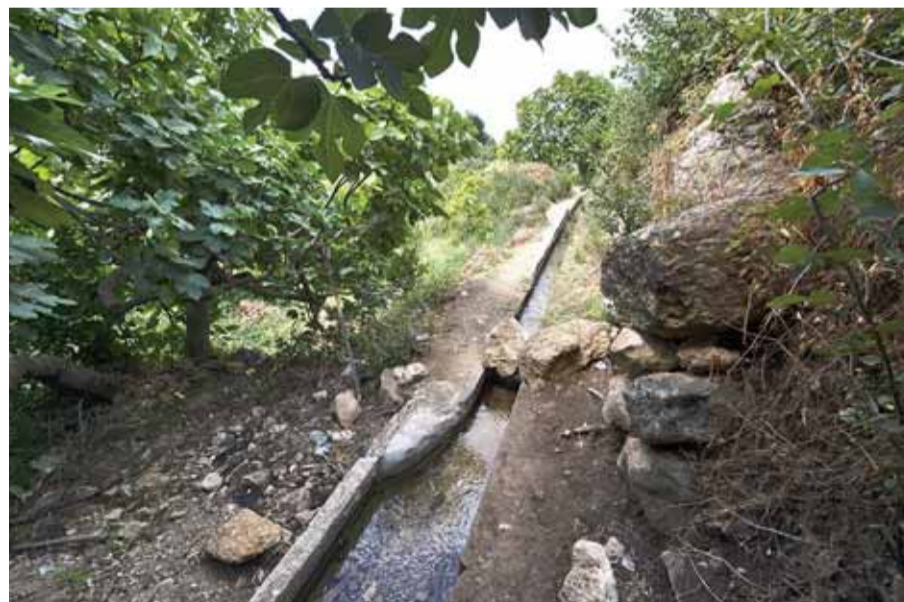
An irrigation system is pictured amidst fig trees in the Tunisian town of Djebba, southwest of the capital Tunis.
