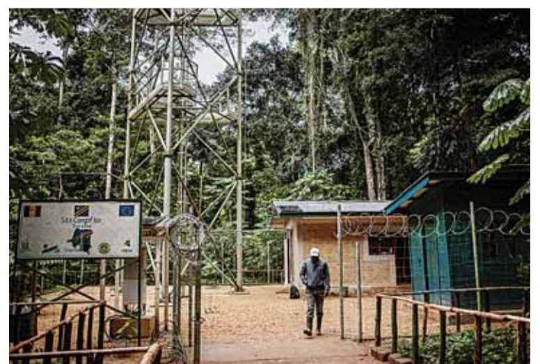
A staff member walks at the base of the Flux tower in Yangambi.
