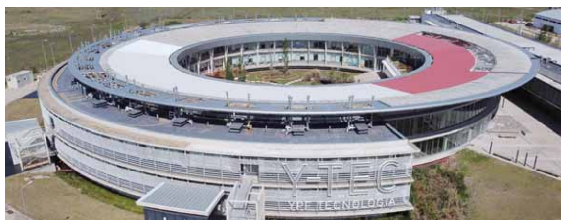
BERISSO, Argentina: Aerial view of the Y-TEC (YPF Tecnologia) headquarters in Berisso, Buenos Aires province. With 19 million tons, Argentina is, after Bolivia, the country with the largest lithium reserves. Now, amid the 'white gold' boom, it wants to control the entire production chain: from extraction in the salt flats to manufacturing electric cars. — AFP
